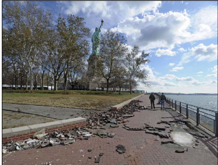
Hurricane Sandy Impacts on Liberty Island
