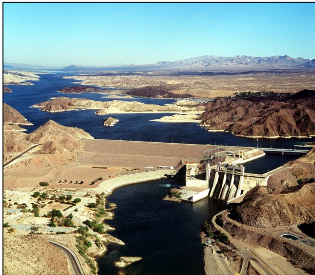
Davis Dam, Nevada and Arizona
